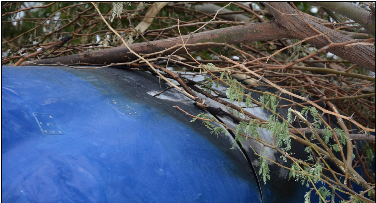
Fig. No. 24: Engine No.1 engine upper cowling exhibiting thermal distress.
